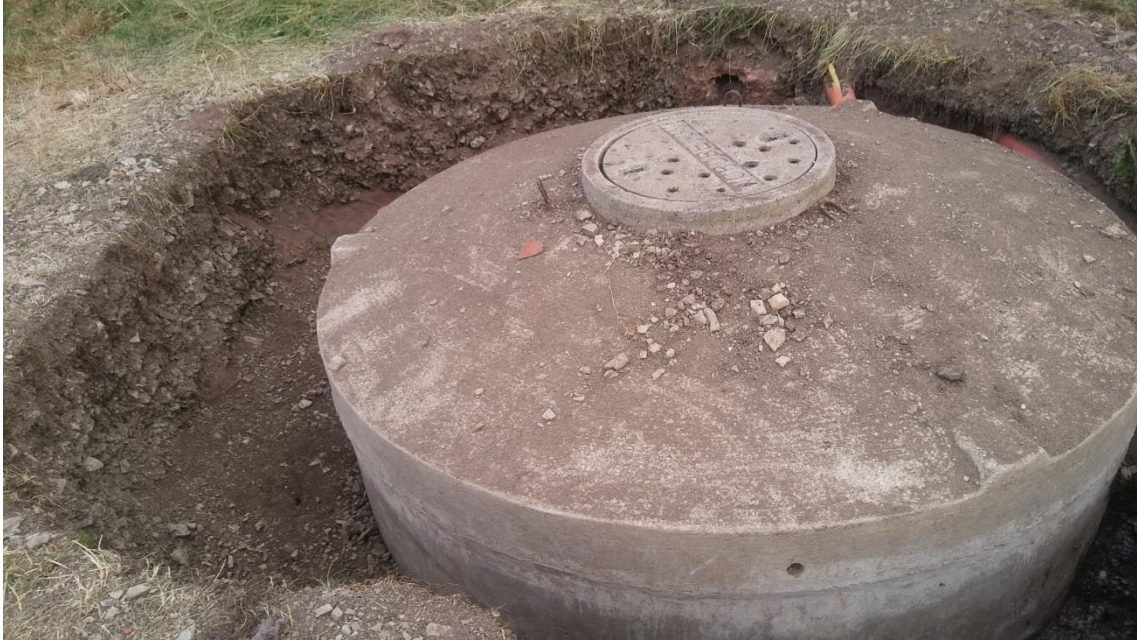
After the first week of "Digging team"
