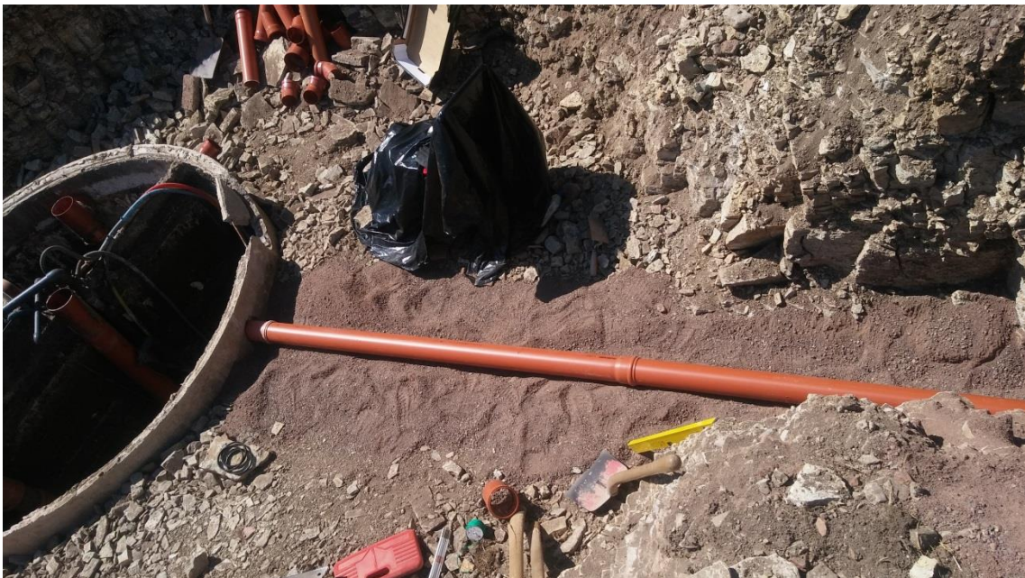
The first pype installed
