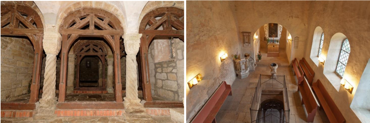
Doppelkapelle interior: on the left, the lower level; on the right, the upper floor
