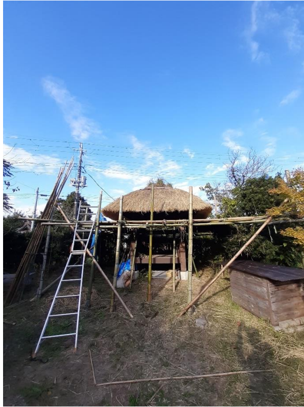
Tetto kayabuki restaurato a Brown's Field
