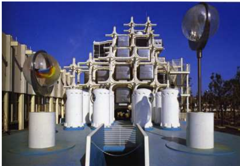
Figure 2.14 Japanese pavilion, designed by architect Kishō Kurokawa at the Osaka World Exposition in 1970.
