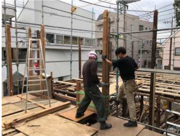
Figure 3.12 Dismantling of Takamizawa house in 2019.
