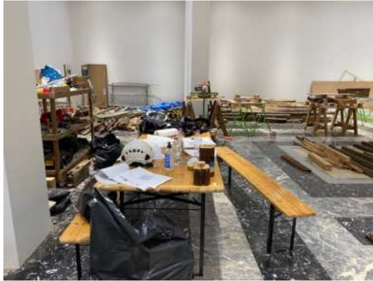
Figure 3.18 Setting up of “Co-ownership of Action: Trajectories of Elements” exhibition at the Japanese pavilion in Giardini di Castello.
