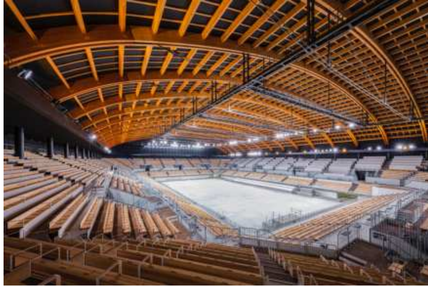
Figure 2.19 Timber Gymnastics Center for Tokyo Olympic Games in 2021: a project by the architectural firm Nikken Sekkei.
