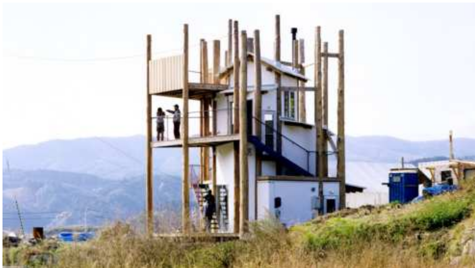
Figure 2.23 “A Home for All” in the city of Rikuzentakata, Japan: a project realized in 2012-2013 by Toyō Itō.
