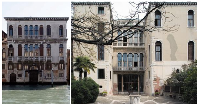
Figure 17 Ca' Tron palace: the facade overlooking the Canal Grande (left) and the internal one on the garden (right) [67].
