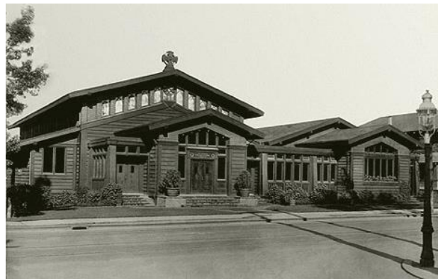
Fig. 71: J. Morgan , St. John's Presbyterian Church, Berkeley, esterno, 1908/1910.
